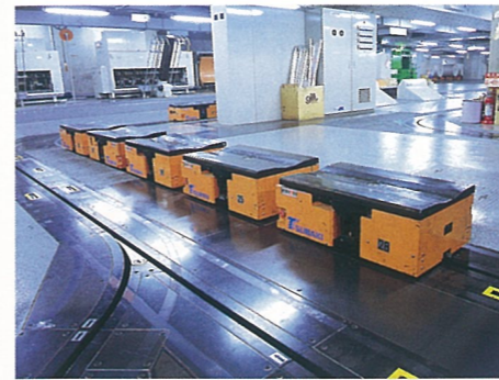
充電待機中のAD AD waiting for battery recharge
