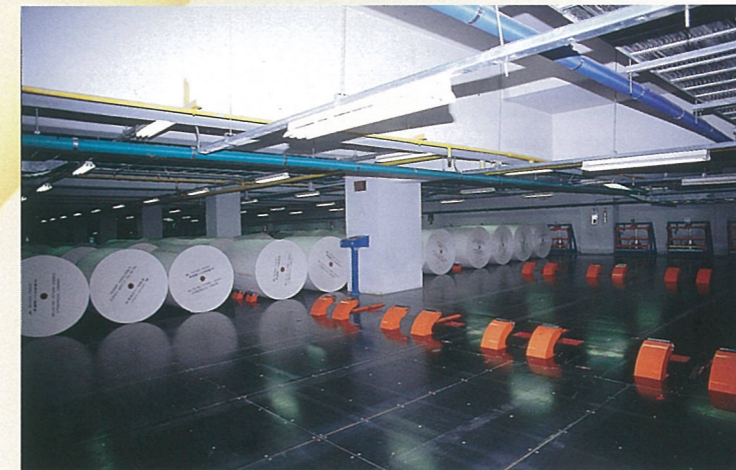
鉄板床 Steel-plate floor
