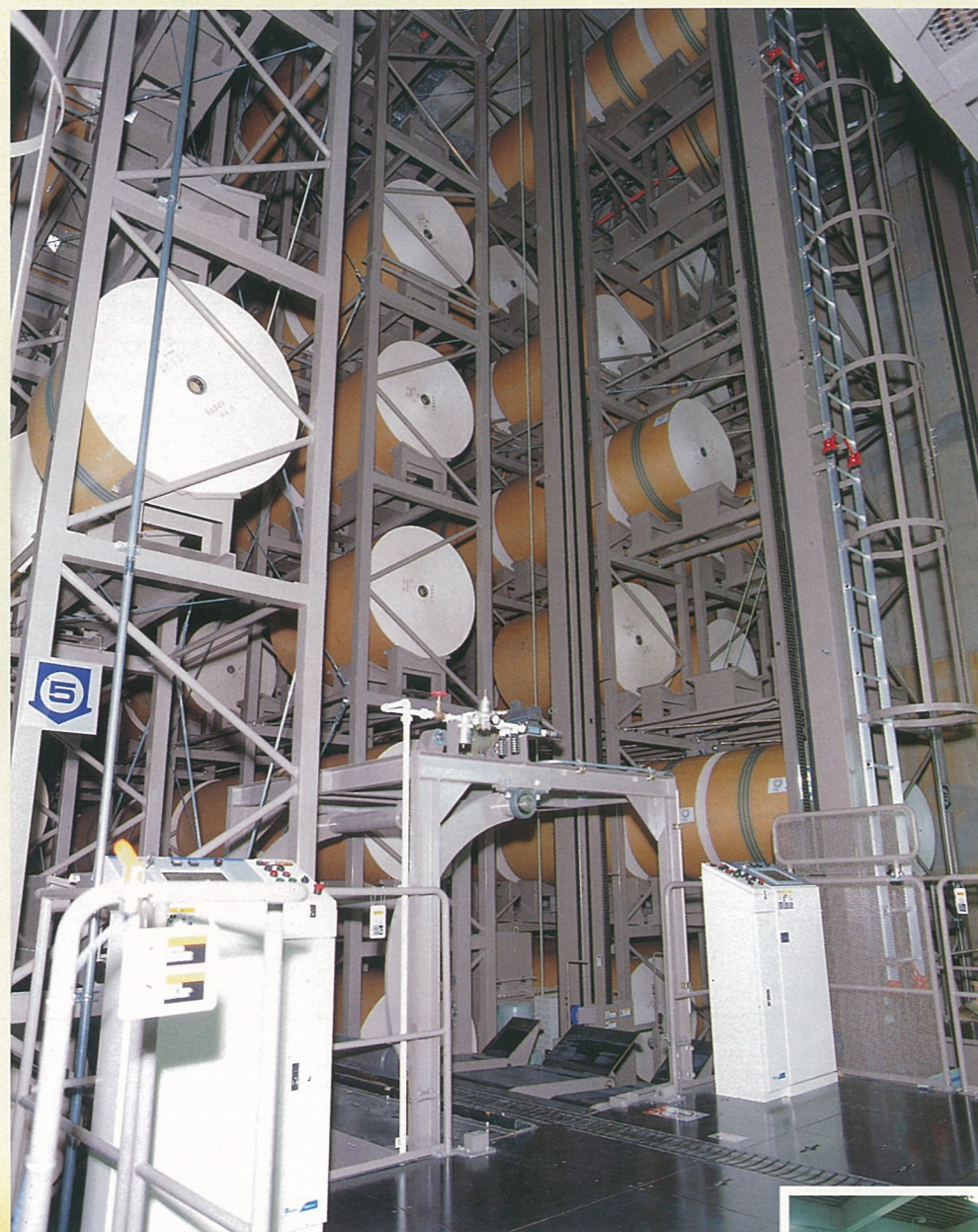
紙庫全景 Overall view of the vertical roll storage yard
